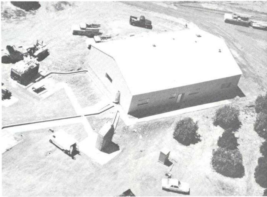
An aerial view of the Santa Paula Station shows the three "troughs" leading out from the control building that will house the electric wiring and waveguide equipment for the three dish antennas. The cement structure in the foreground is the base for the station's 34-foot tracking, command and monitoring antenna.
