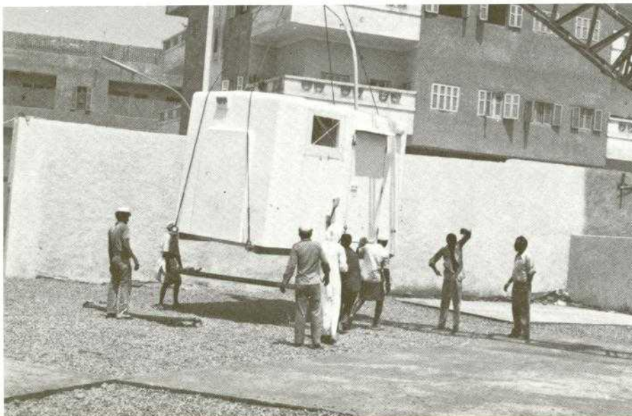
The electronic equipment shelter is off-loaded at the Jeddah site.
