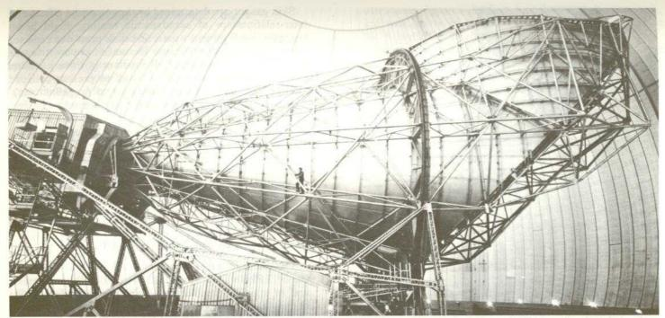
The big horn antenna at Andover, which was used for the first experimental satellite transmissions via Telstar, is scheduled to be replaced in 1971 by an updated 'wheel and track' antenna equipped with a reflector 97 feet in diameter or larger. The horn antenna has been a tourist attraction in Maine since it was built in 1962.
