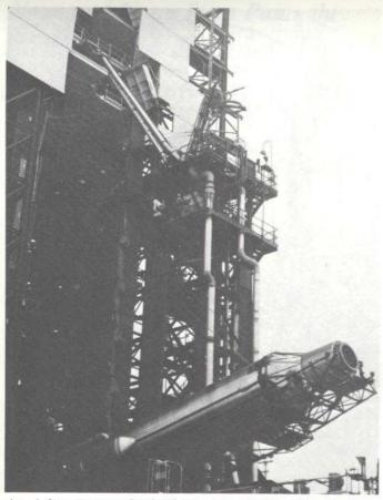
An Atlas stage-and-a-half booster of the Atlas-Centaur launch vehicle to be used in lifting the INTELSAT IV communications satellite into space is erected at Complex 36A at Cape Kennedy, Florida.
